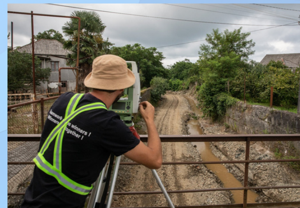
Collecting risk data for rehabilitation of a water channel
