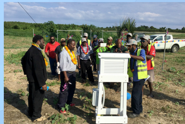
Newly installed weather station © UNDP Vanuatu
