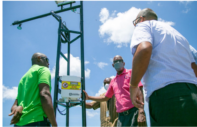
UNDP/ Barbados - installing early warning signal
