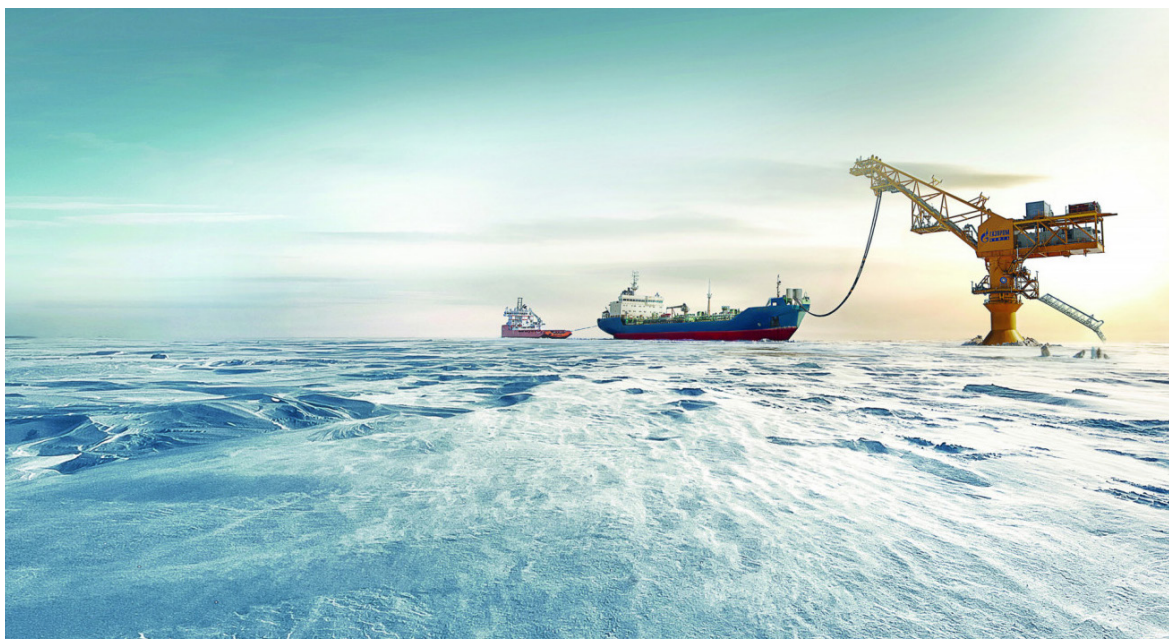
» The energy industry and foreign investors demanded huge tax breaks to launch production facilities in Russia's arctic. © gazprom-neft.ru
