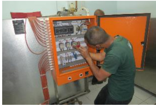
Tightening the screws of the JSD 1300 contactors
