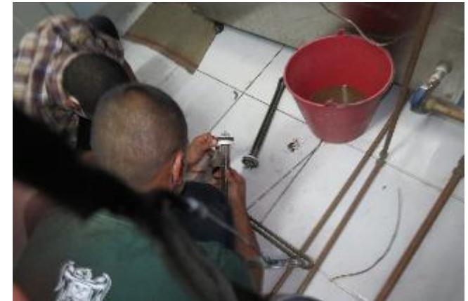
Checking, replacement of a JSD 1300 element
