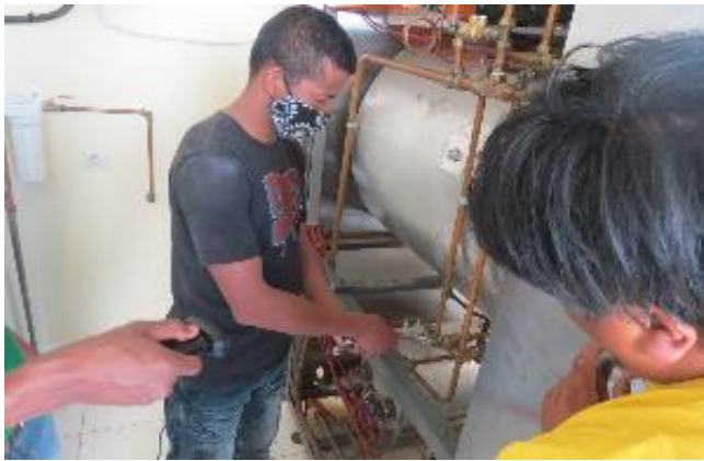
Replacing a JSD 260 valve
