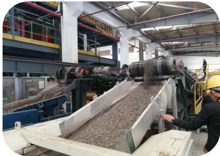
Bottom ash sorting equipment
