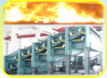
Incineration and heat recovery boiler system
